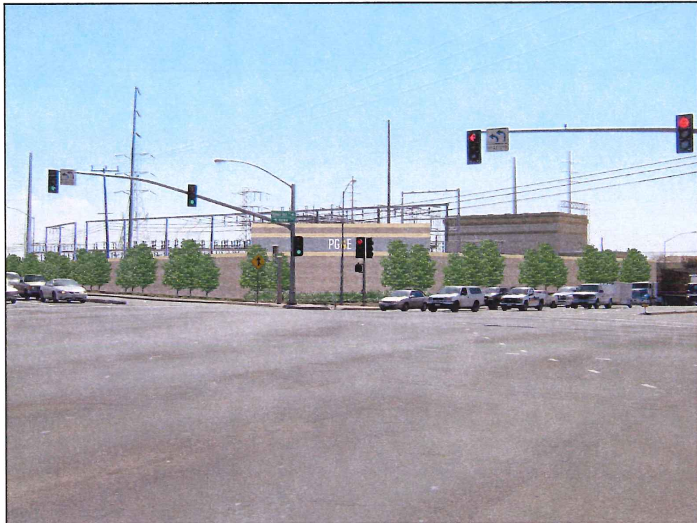
PG&E Substation Screen Wall
