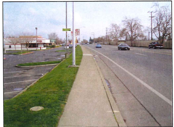
Existing Sidewalk at Raley's Shopping Center
