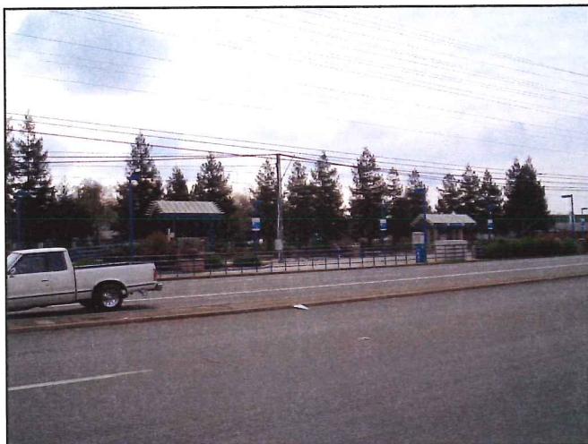
College Green LRT Station
